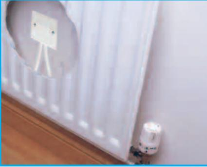
The pipes exit a single gang box (fitted with rubber grommets) located at the mid height of the finished radiator position. This also provides a fixed point for other trades to work to and reduces the risk of damage to the pipework.
