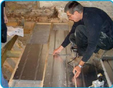
Spreader plates 390mm x 1000mm are designed for use with traditional joists at 400mm centres. They are laid across the top of joists and fixed in place using a hand stapler.
