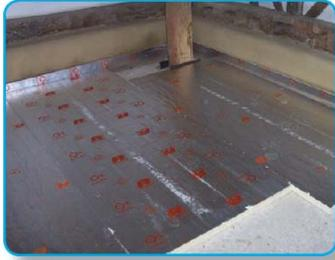
Make sure the floor is cleared of dust and debris. Lay the floor insulation and edge insulation and tape all joints to prevent the ingress of the screed.
