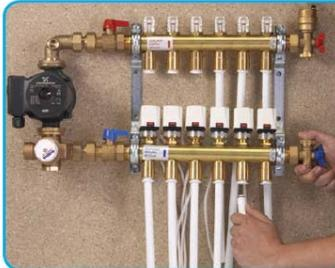
The Speedfit pipe can now be connected to the manifold.
