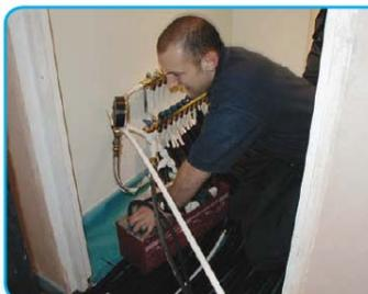
The system can now be filled with water and pressure tested using correct methods.
