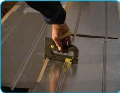
The Speedfit pipe is pushed into plates grooves at a fixed 200mm centres. The joists will need to be notched at one end to continue the circuit and return to the manifold.
