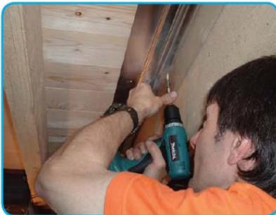
Spreader plates 165mm x 1000mm are designed for use with either traditional or TJI joists where the finished flooring is already in place. They are fixed to the flooring from underneath using either screws or staples.
