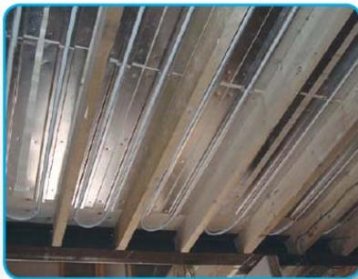
They can also be used on either 400mm or 600mm centre joists. The Speedfit pipe is pushed into the plates grooves from underneath at a fixed 200mm centres. Insulation is then placed between the joists to the underside of the plates.
