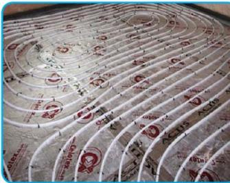
The Speedfit pipe can now be laid in a pre-determined pattern and fixed to the insulation with either Pipe Staples or Clip Rail.
