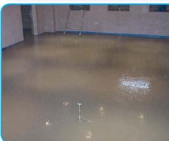
The system can now be screeded. The system should remain under pressure until the screed has cured. Do not use the system to dry the screed.
