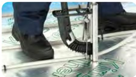
The pipe should be installed at 200mm centres.
