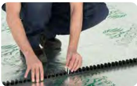
Continue to fit the clip rail across the room at 1m intervals making sure that sufficient space is left around the perimeters of the room (approx. 800mm) to accommodate any pipe returns or connection lengths back to the manifold. Care should also be taken to ensure that the clipping alignment is maintained.
