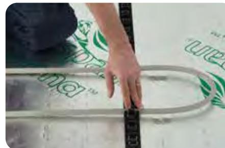
Continue to lay the pipe in this serpentine pattern until you have reached the end of the circuit.
