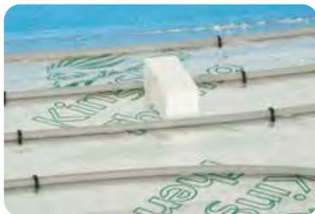
The plastic skirt should be laid over the insulation and the outside run of pipe stapled into the skirt covered insulation to create a seal around the edge of the area.
