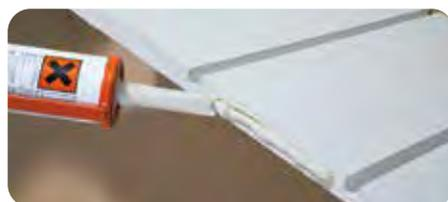
When gluing the ends, ensure there is no residual glue in the pipe grooves and use short lengths of pipe to help with panel alignment.
