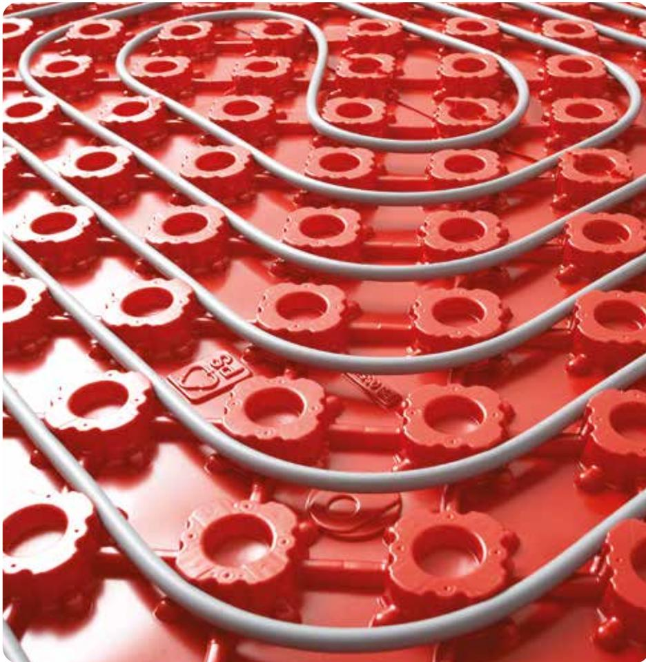
**Panels step 6: Laying the pipe**
